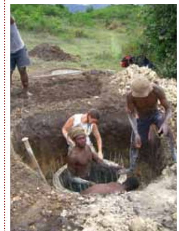
Working hard digging a well in Madagascar
